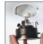
Insert trim to complete installation.
