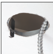
Support clip keeps plaster frame in place during rest of installation.
