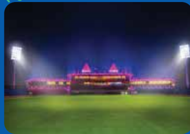
Situated at an altitude of 1,457 m above the sea level, we illuminated HPCA, the international cricket stadium in Dharamshala, with 384 Philips Sportsar and DMX lighting controls.
