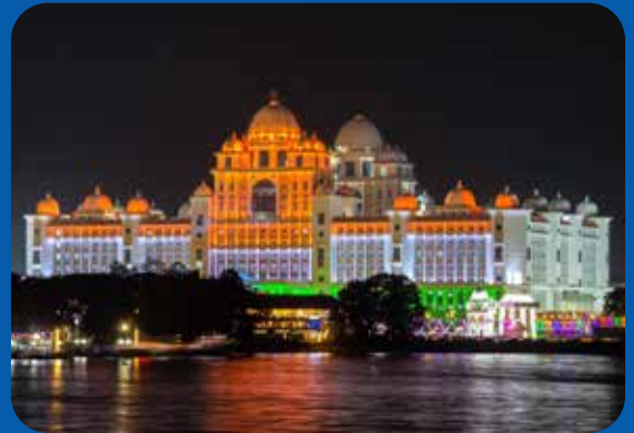
We illuminated iconic facade of Telangana Secretariat making it a visual masterpiece for both day and night.
