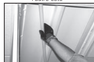
Figure 8. Installation des lampes
