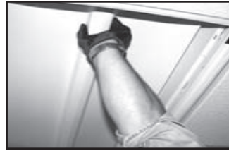
Figure 7. Squeeze and Install Opposite Side
