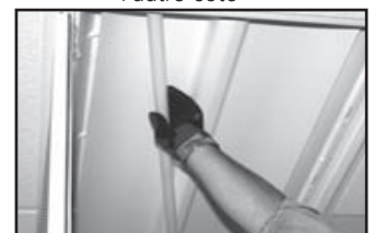
Figure 8. Installation des lampes
