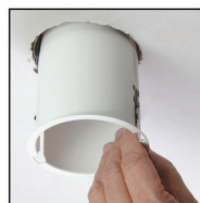
Insert housing into position and align slots in housing wall with indicator label on inside of plaster frame opening. Then secure in position with cam locks.
