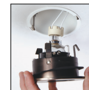
Insert trim to complete installation.
